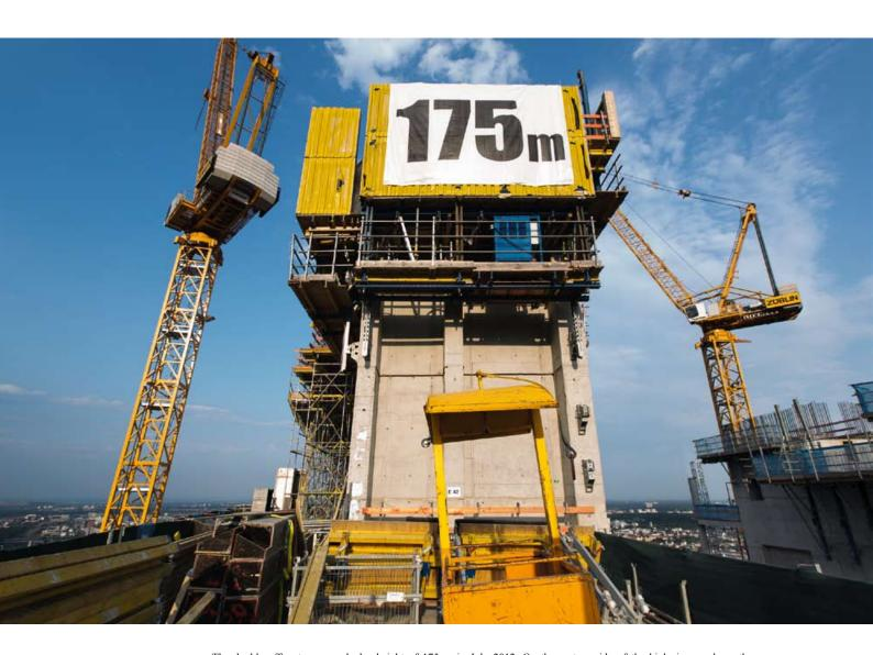
The double office tower reached a height of 175 m in July 2012. On the eastern side of the high-rise, work on the construction of the framework for the glazing of the atrium is under way.
