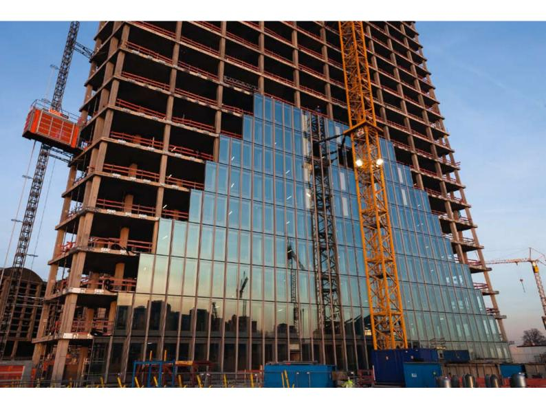
The mounting of the energy-efficient facade panels for the double office tower began in February 2012 and is continuing alongside the fit-out works and the installation of the technical infrastructure. The facade has a grey, non-mirror finish with a light green sheen so that it blends into the surrounding environment.
