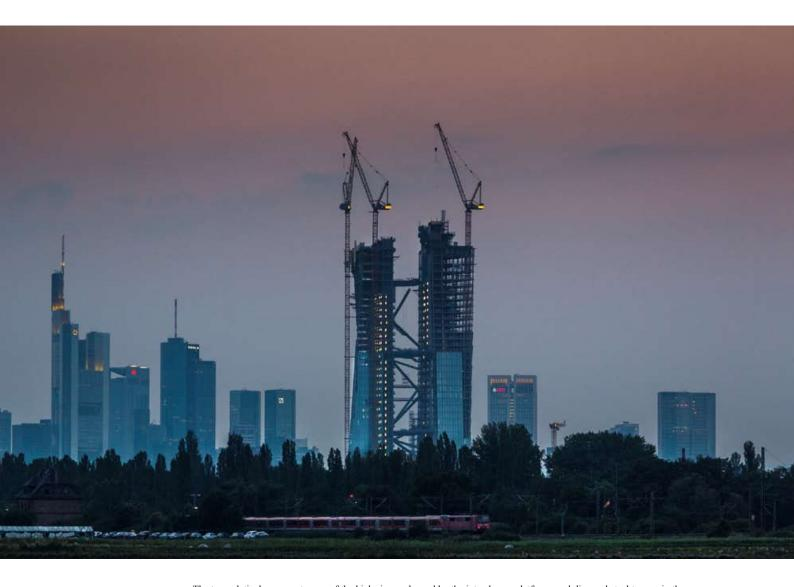
The two relatively narrow towers of the high-rise are braced by the interchange platforms and diagonal steel trusses in the atrium. The various platforms and steel structures within the atrium were completed in November and December 2012.
