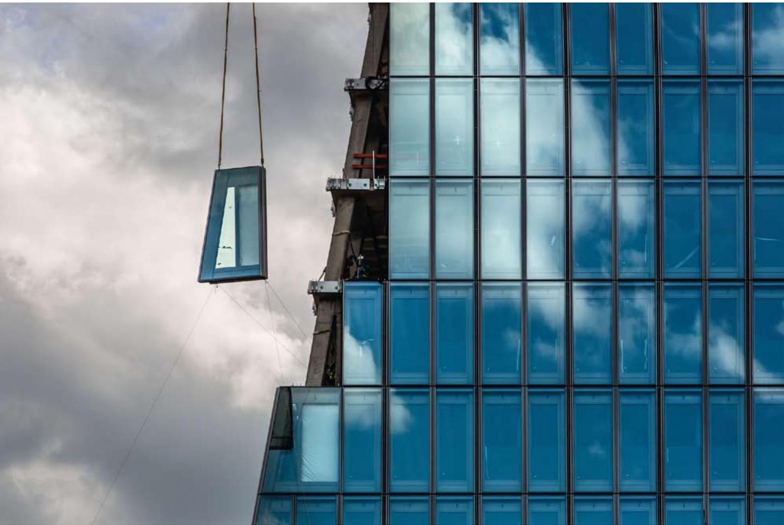
By September 2012 approximately two-thirds of the facade and the main structural works had been completed, so that the final look of the double office tower became easy to visualise. The deconstructivist design of the building means that it looks different from every angle. The height of its structural framework is such that the torsion of the southern and northern facades, i.e. the twisting along the longitudinal axis, is clearly evident.
