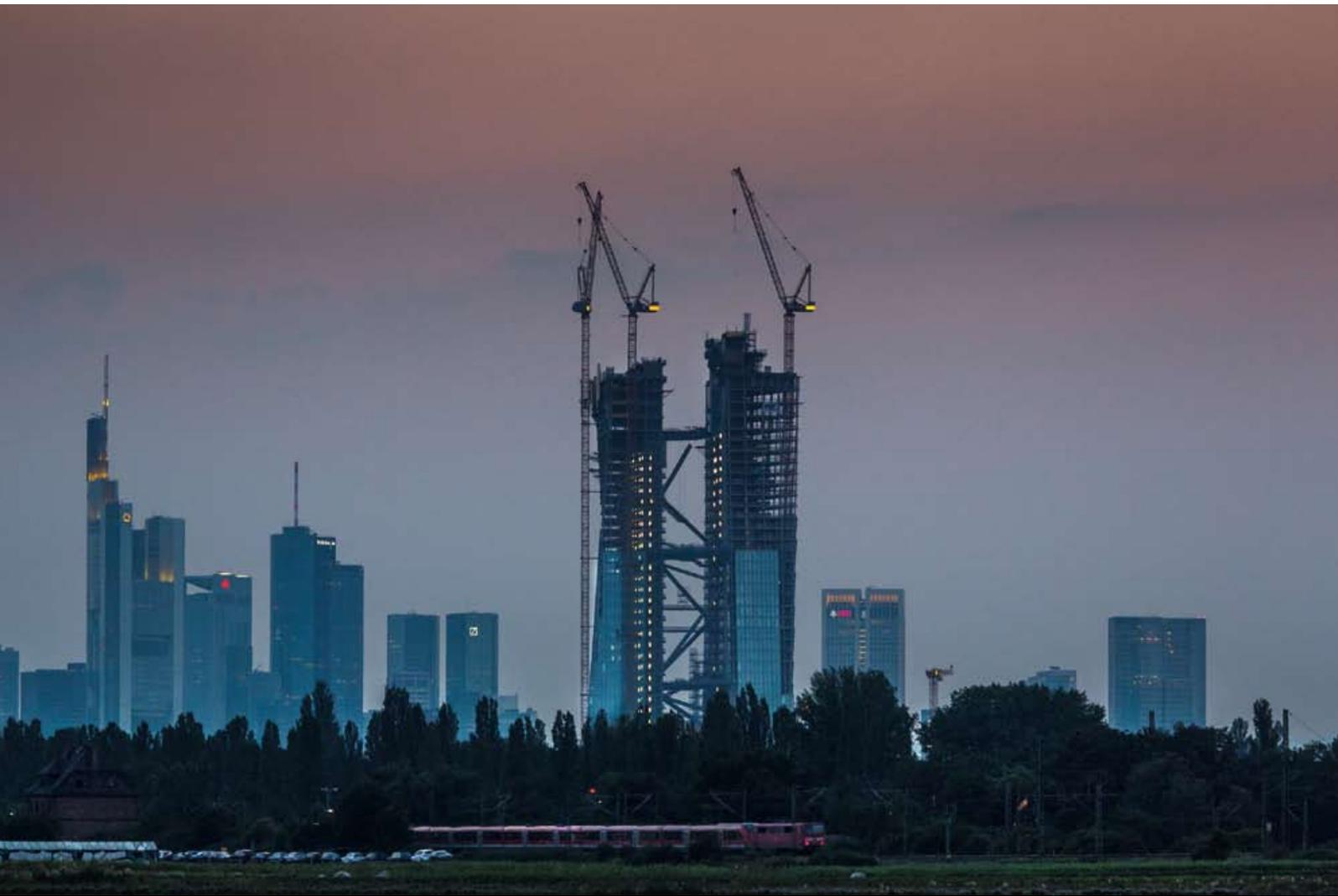
The two relatively narrow towers of the high-rise are braced by the interchange platforms and diagonal steel trusses in the atrium. The various platforms and steel structures within the atrium were completed in November and December 2012.
